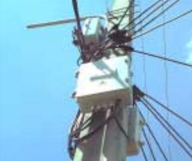
*The meters are installed outside the house in a pole-top box. This makes it almost impossible for a person to open the box and tamper with the meter.*
